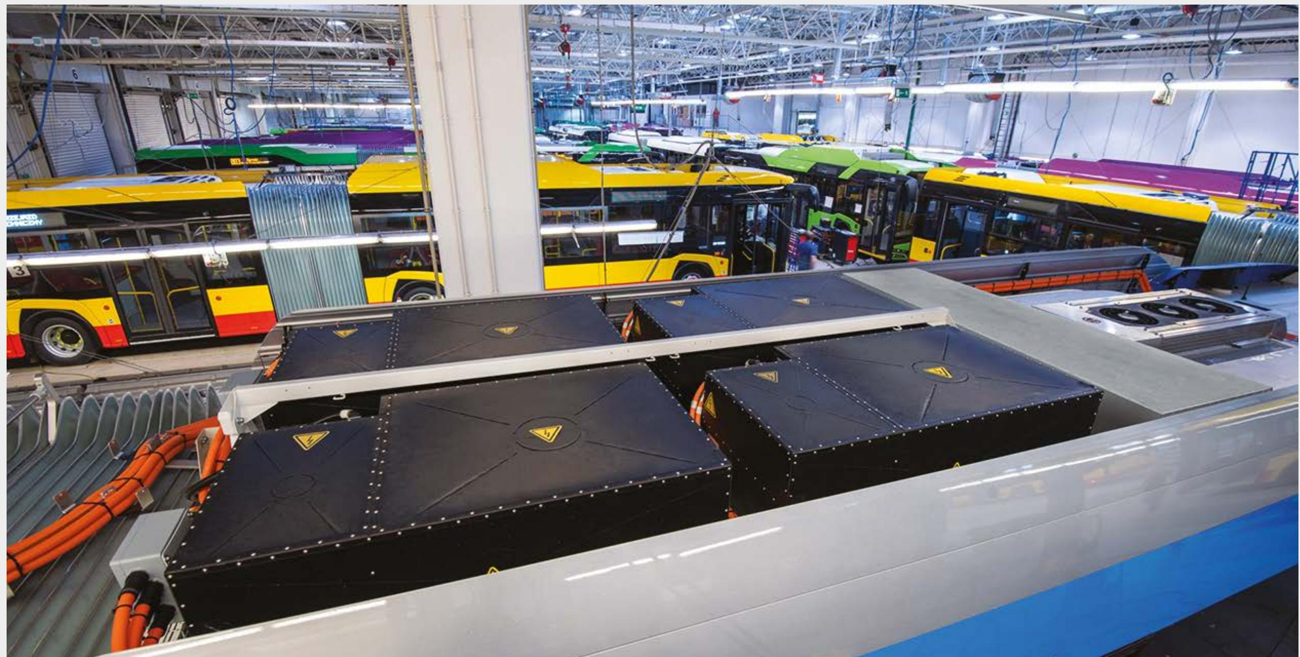
Batteries that, over time and as a result of their operation, have run down their capacity can still serve as an excellent form of electrical energy storage in stationary applications. This is the inspiration behind the idea for the second-life battery project, which Solaris will implement in cooperation with TAURON and Impact.
